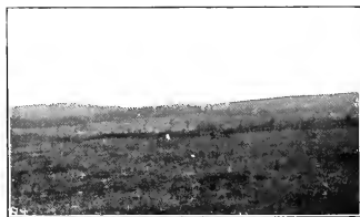
Wire entanglement near Boureuilles, through which the 110th Infantry advanced in Argonne Drive.
